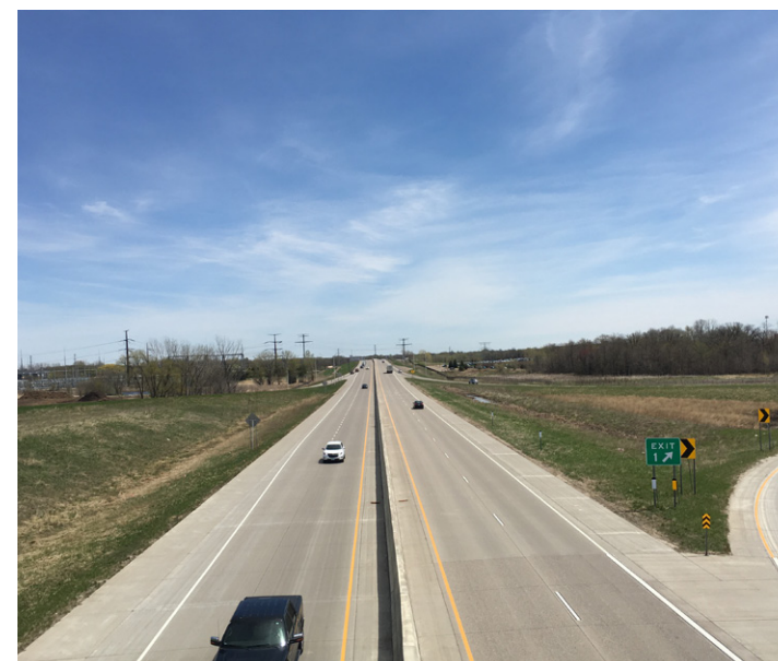
State Highway 610 existing conditions
