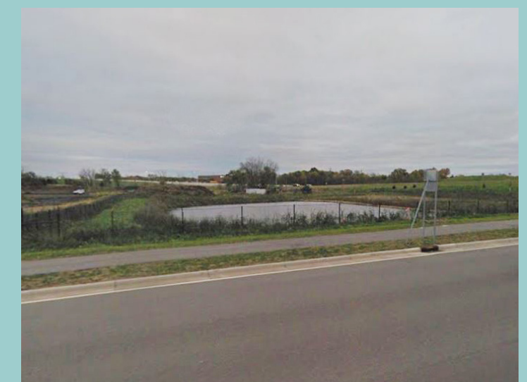
Existing stormwater pond
